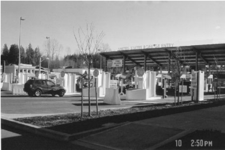
Fig. 10.34 Sensitive monitors installed at portals in passenger lanes of border crossings into the U.S. can detect small amounts of radioactive material. Alarms are sometimes triggered by naturally radioactive agricultural products, ceramic tiles, and occasionally by a passenger, recently administered radioactive
